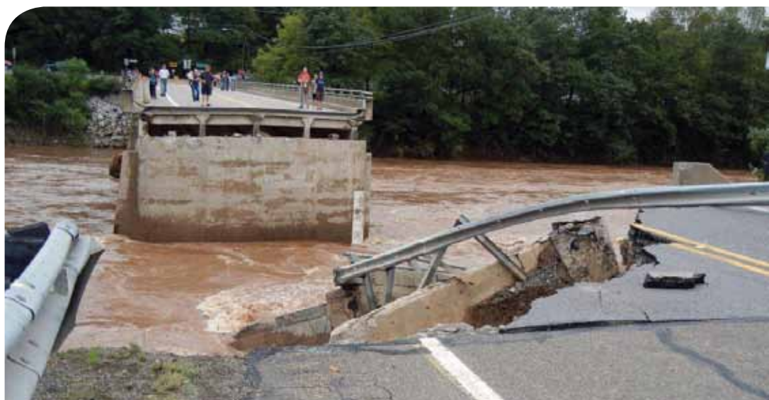
This bridge in Lycoming County was completely washed out by Mother Nature’s fury.
