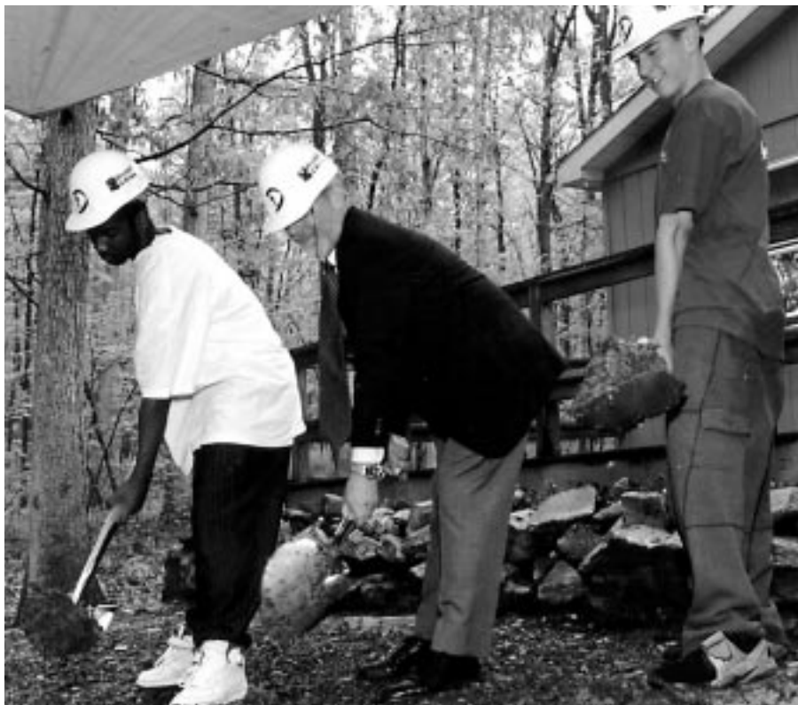
Breaking ground for the Wilderness Center's expansion are, from left to right, current student Jason Kissinger of Reading, Executive Director of the center George Eckenrode, and Hosea Twiggs of Philadelphia, a former student.
